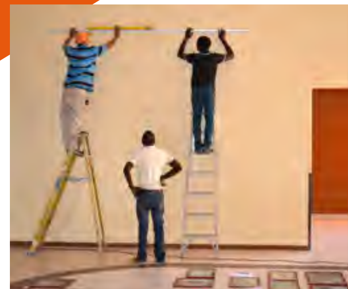
The hanging system was professionally installed. Whilst time-consuming it is very important that the rails are level and at a suitable height.
